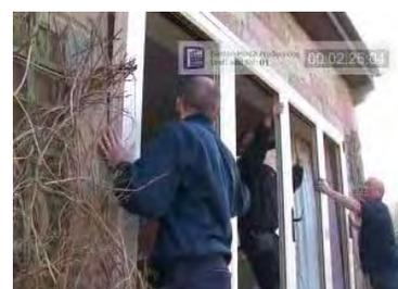
Once in the correct position and the door is plumb and square without twist, you can begin fixing the door into the opening, using appropriate fixings (not supplied). When fixing down to the cill, ensure that screws are sealed to prevent water ingress. Also seal across the cill below the door jambs to prevent water tracking across the cill.
